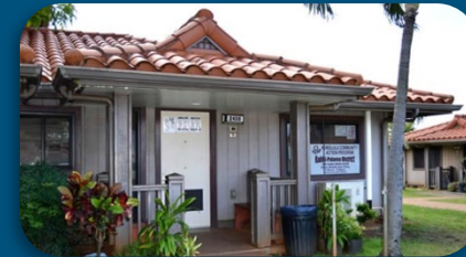
Kalihi-Palama District Service Center
